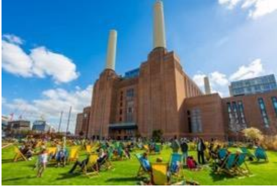
Battersea Power Station, (BPS) UK
